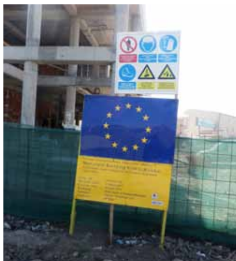
Construction of Kllokot/Klokot Municipality
