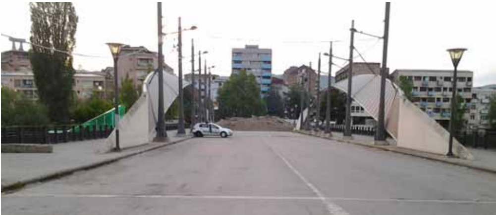
Barricade on the bridge over Ibar river
